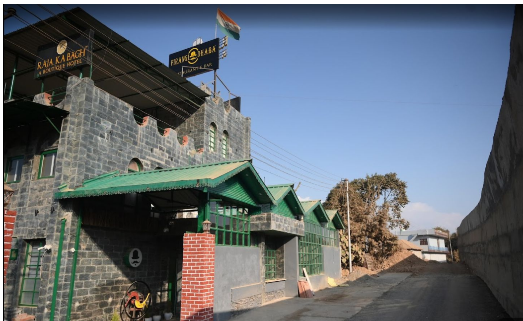
Side elevation with Firangi Dhaba signage above — visible to highway traffic from both directions.
