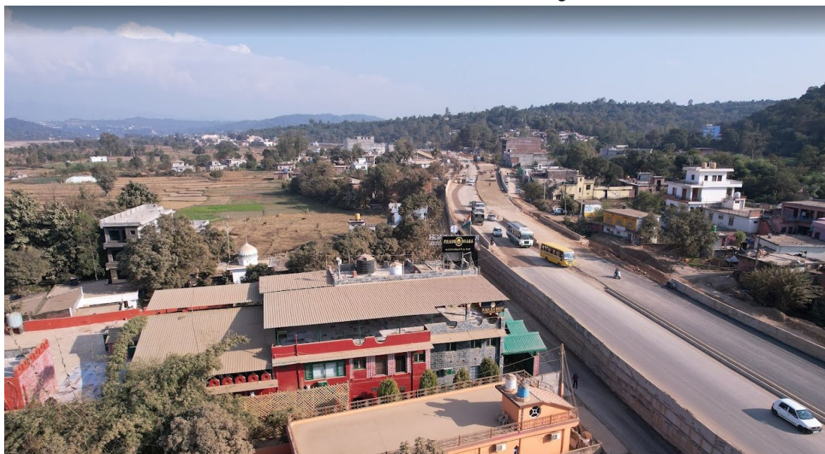
Aerial view — property fronting NH154 (Pathankot–Mandi 4-lane). Median exit visible.
